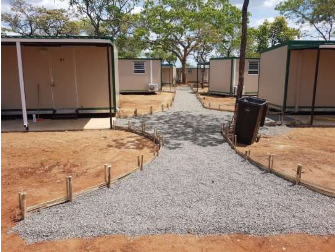
Figure 3: Camp accommodation complete
