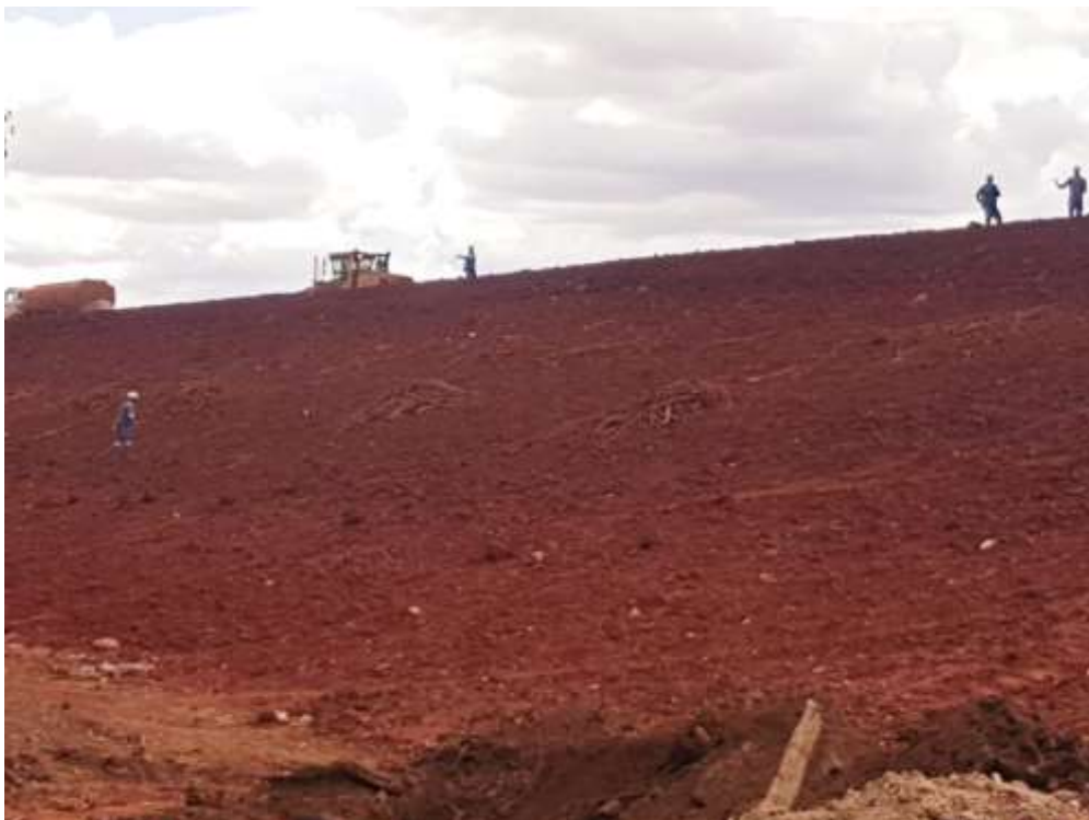
Figure 2: Tailings Storage Facility wall complete
