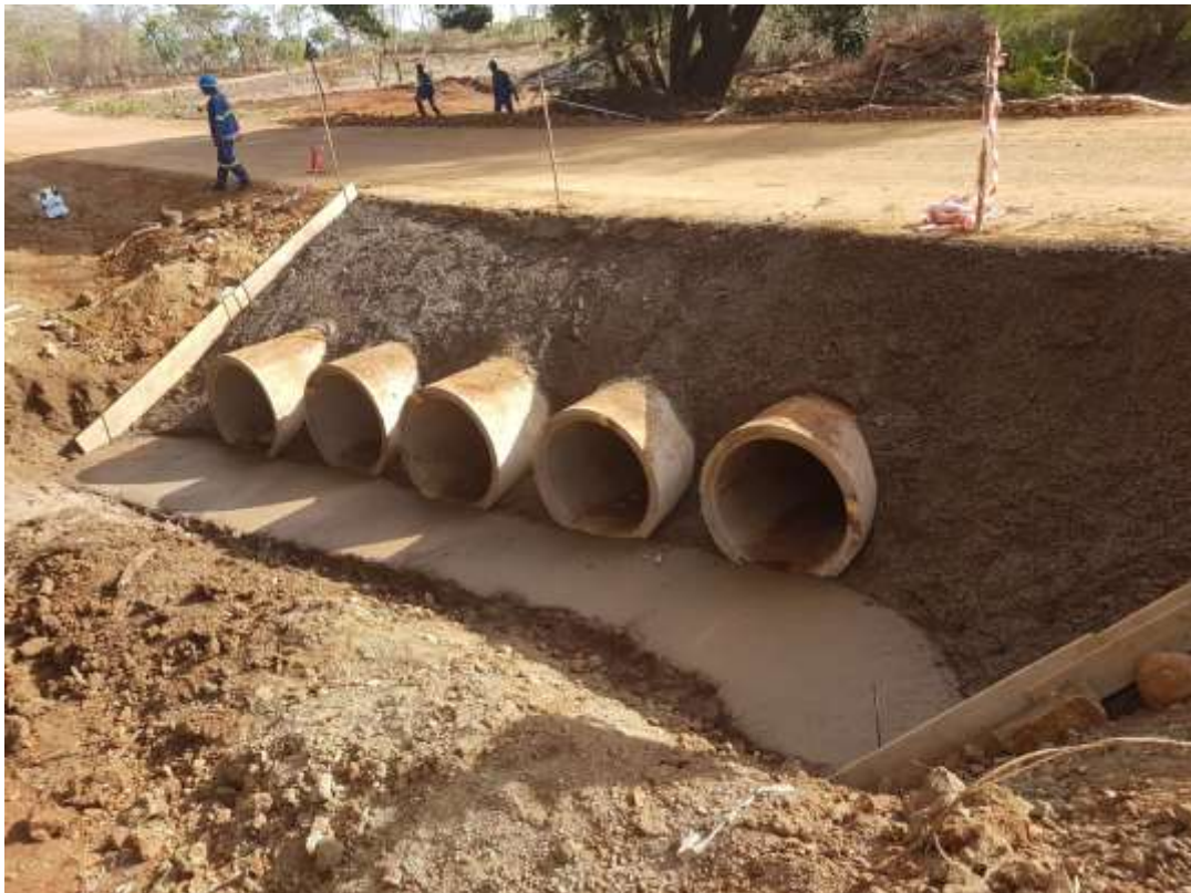
Figure 4: Access Road Culvert Construction
